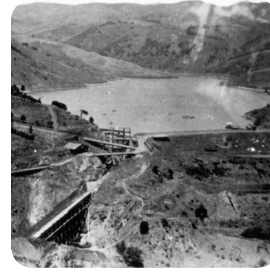
In the 1870s, not long after California became an American state, Lake Chabot was built by Chinese laborers living at Camp Yama-Po, using a dam on San Leandro Creek. The lake provided water for agriculture and growing towns.
